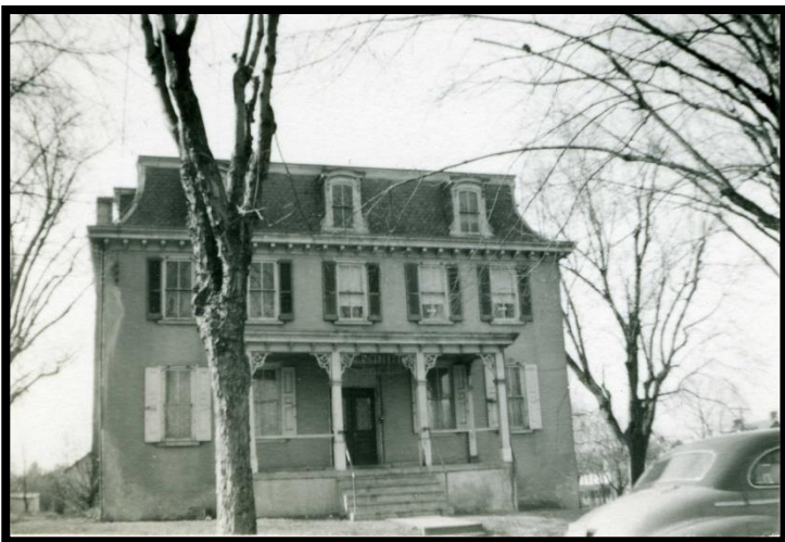
5. North Wales Legion Demolished 1964
